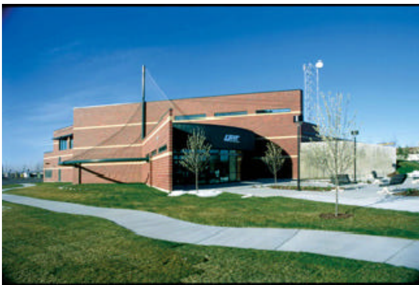
The UDOT Traffic Operations Center serves as the hub for Department of Public Safety dispatchers and TOC operators.
