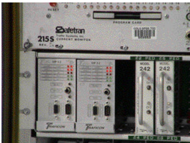
View of video image process (VIP) inside a cabinet.
